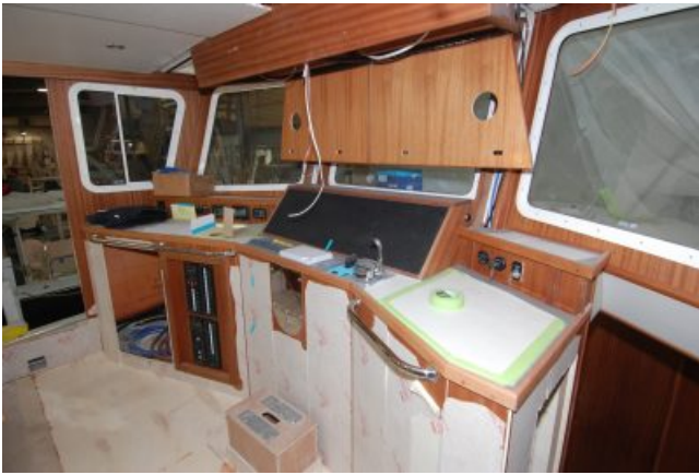
Pilothouse is coming together nicely.
