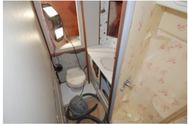
2nd stateroom head almost done.
