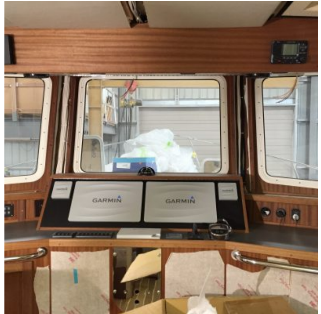
Electronics are now installed. 2, 16" Garmin chart plotters, Garmin autopilot, Meratron monitoring system, Icom VHF with class B AIS, Cummins engine management system, Garmin GMI20
