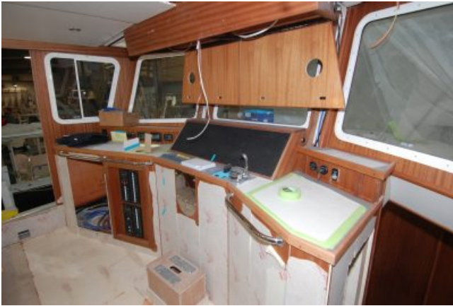
Pilothouse is coming together nicely.
