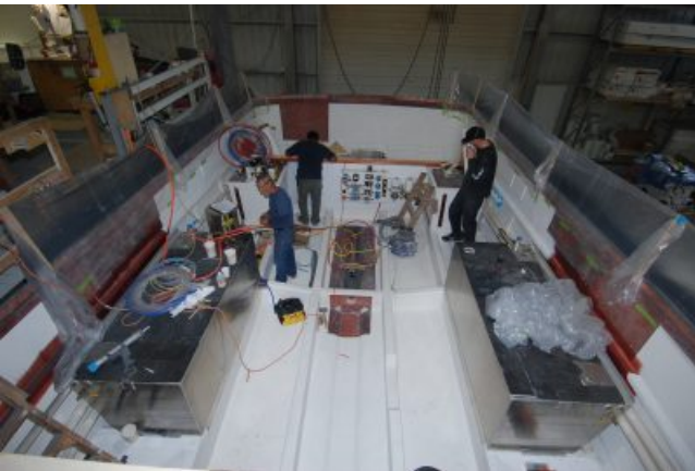
All the major mechanical and most of the wiring must go in before the deck goes on. In this picture you can see the fuel tanks on both sides. They are 320 gallons each for a total capacity of 640 gallons.
