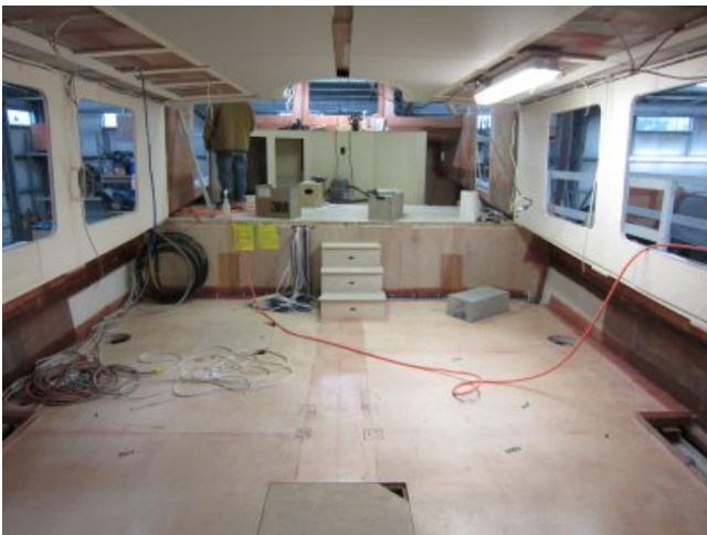
This picture shows the salon area looking up into the pilothouse
